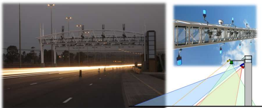
Figure 4: ORT: The Gantry Source: ETC (2010)
