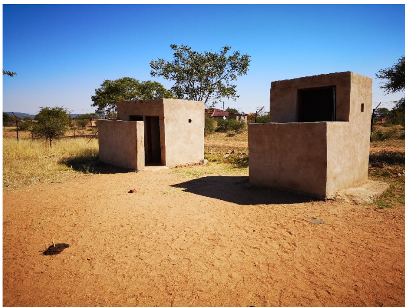
Figure 3.1: Old toilets at Ncheleleng Secondary School
